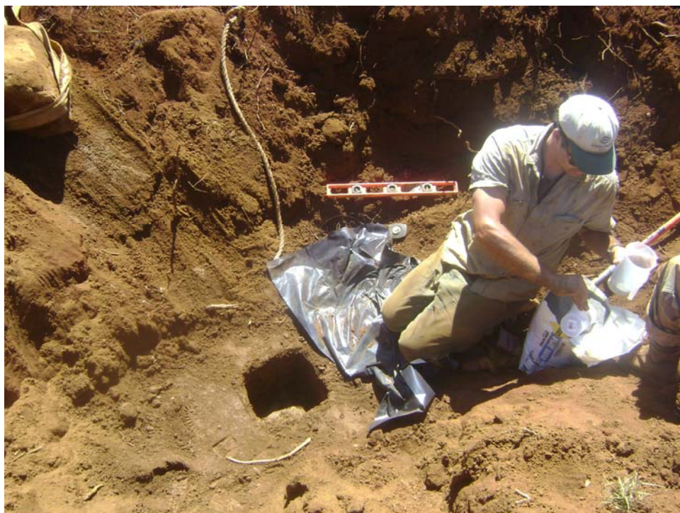
Trench no. 1 – Density sample
