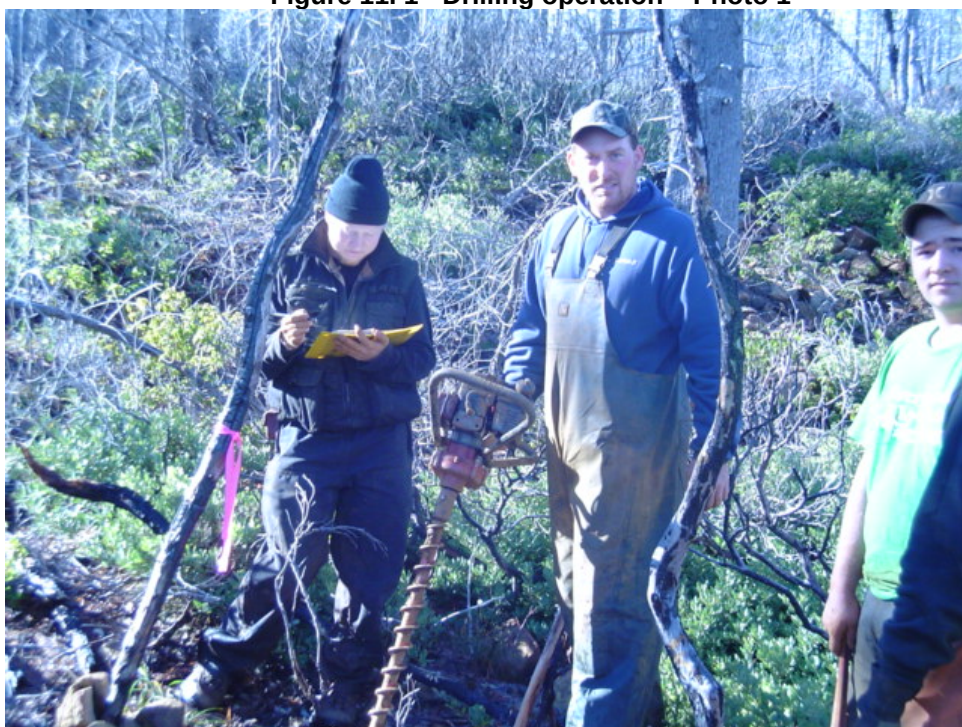
Figure 11. 2 - Drilling operation – Photo 2
