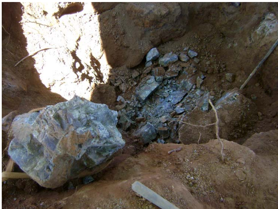
Trench no. 5 – Rock (4ft)
