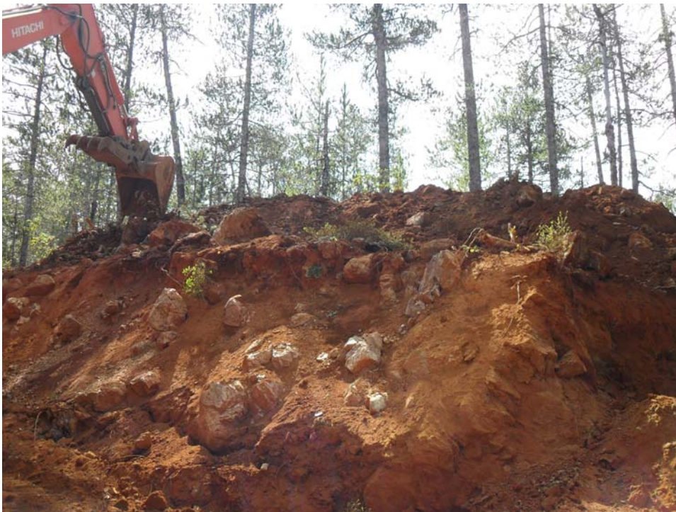
Excavated soil and rocks from trench no.4
