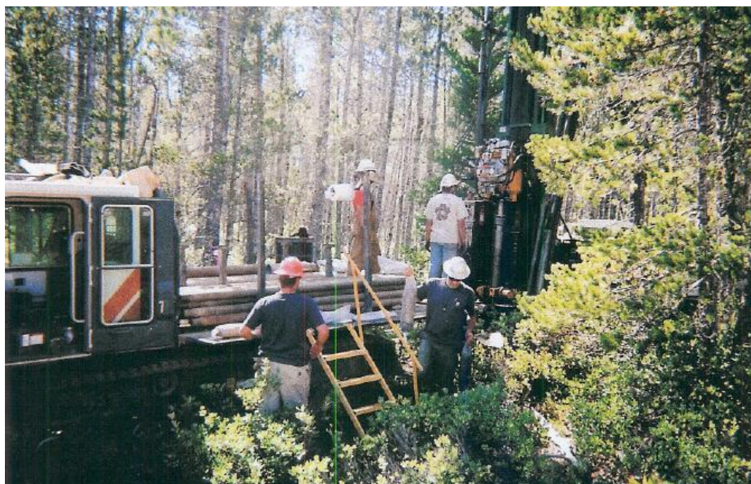
Figure 11. 1 - Sonic drilling operation
