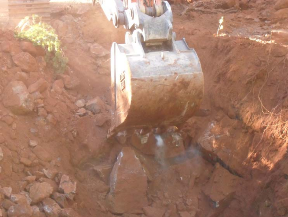
Excavator digging – trench no. 1
